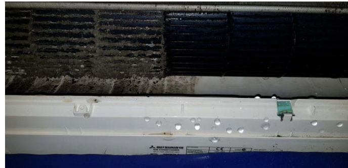
Photo – Before & After Clean
